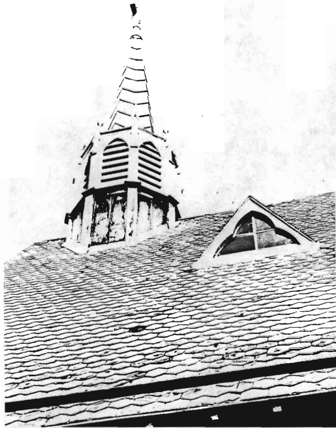
Roof and belfry detail.
