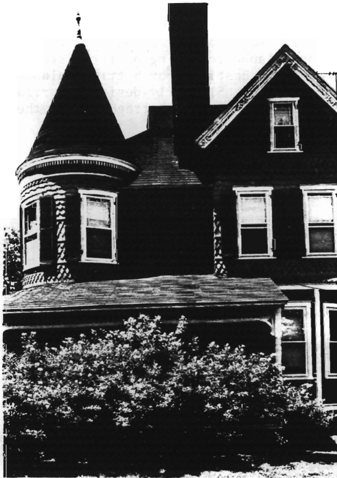
Detail, east facade.
