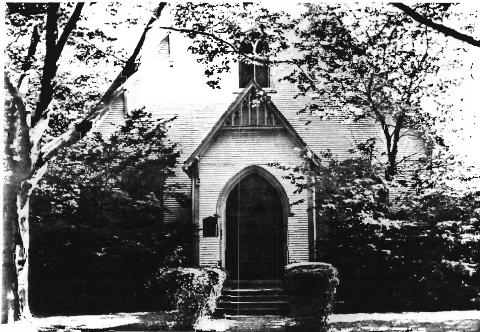
Main facade detail.
