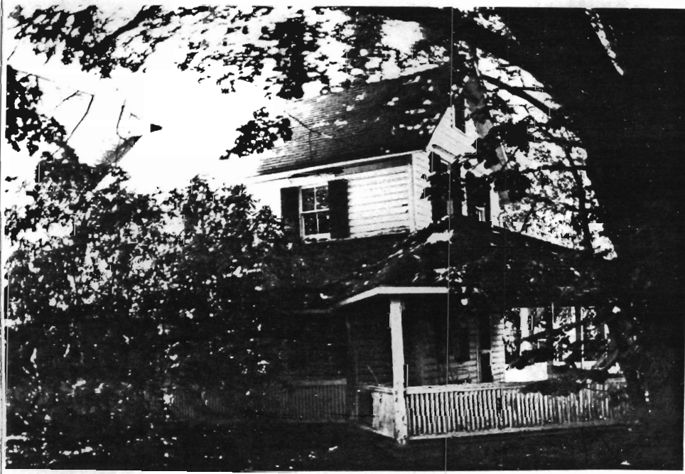
East wing, view south. (Heavy overgrown vegetation makes site difficult to photograph)
